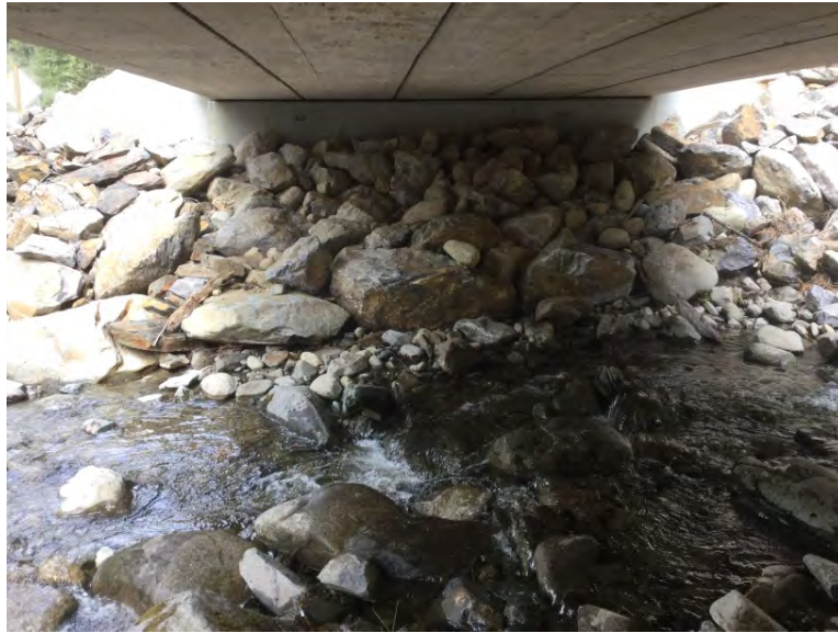
Right Bank Abutment when facing downstream
