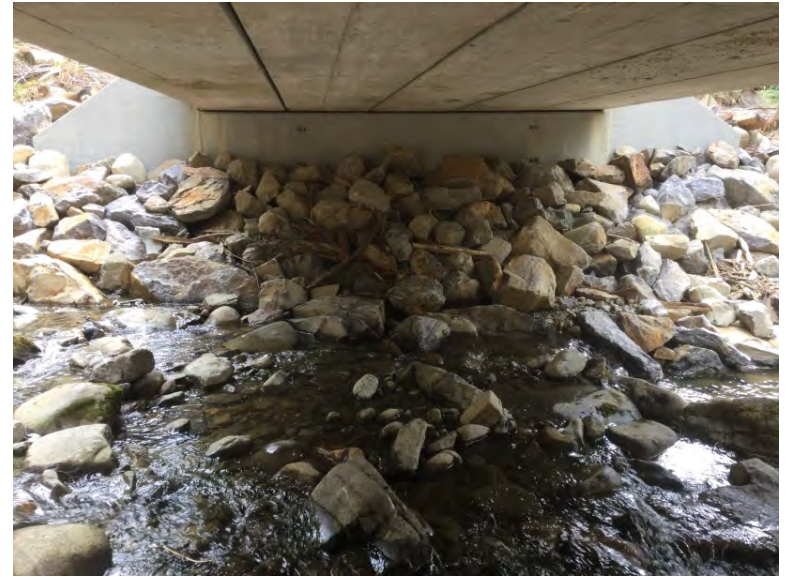
Left Bank Abutment when facing downstream
